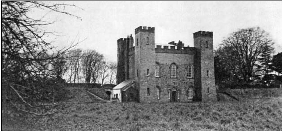
Photograph of Hillsborough Fort in the 1950s, clad in slates. The walls and towers were originally rendered, but in the late 19th century were clad in slates in efforts to keep out the damp. The building was re-rendered in the 1980s for similar reasons.
