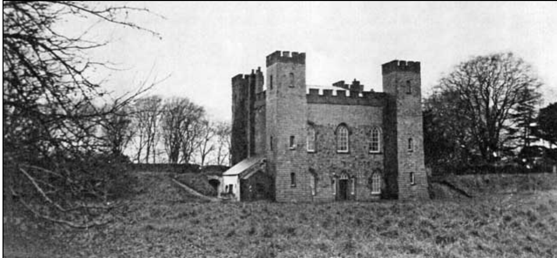
Photograph of Hillsborough Fort in the 1950s, clad in slates. The walls and towers were originally rendered, but in the late 19th century were clad in slates in efforts to keep out the damp. The building was re-rendered in the 1980s for similar reasons.
